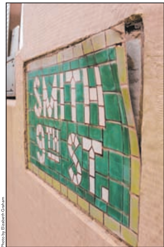
Most of the mosaics at the Smith-Ninth station are made of paper — and this one is peeling off.
