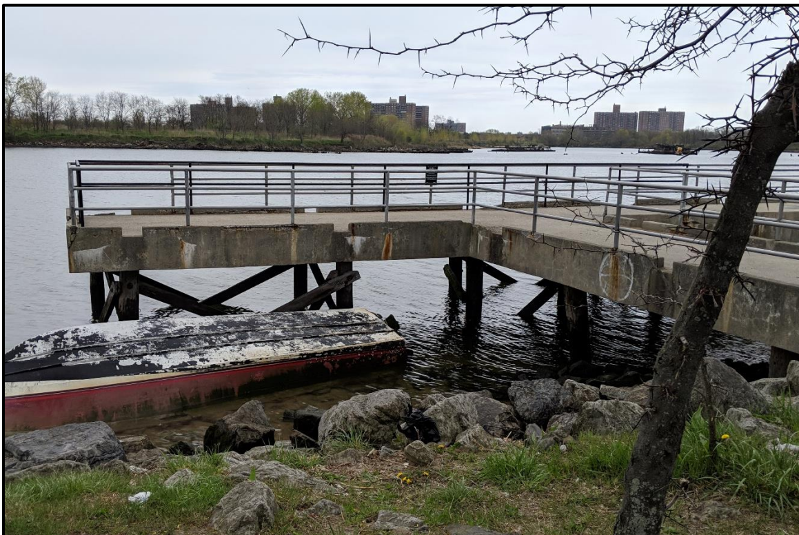
PHOTO 4: View of the existing pier at the location of the proposed landing, looking north.
