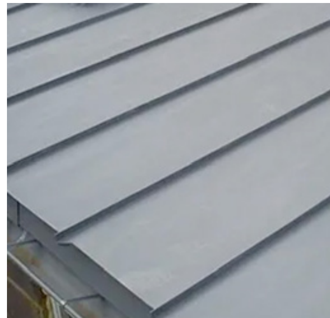
Standing seam zinc roofing
