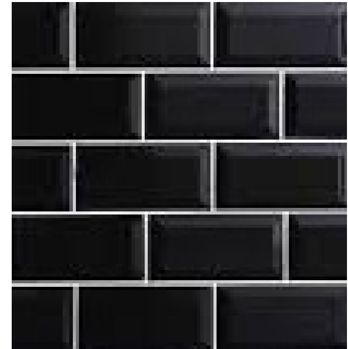
Internal tiled walls
