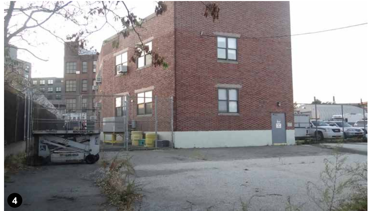
Southeast view of existing ERU building.
